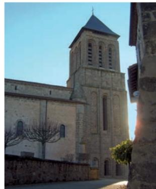
The north and south elevations are supported by flat buttresses. These buttresses mark the spans. Each bay is pierced to the north and south of a semi-circular bay. The nave, which is higher, projects beyond the side aisles. It has small rectangular openings under the cornice. The semicircular apse is pierced with three semicircular bays. Two flat buttresses support the walls between the bays.
