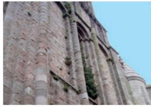
The companions of Saint James from Barbezieux were responsible for restoring the masonry and replacing the stones that were too damaged. The rammed earth of the forecourt was also reworked to give it a more uniform appearance. The slate roof was completely relaid. It was surmounted by a new copper cockerel.
