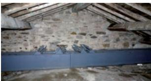
The tie rods are placed on three transverse arches, with four tie rods per arch : two at the connection between the nave and the aisles and two on the exterior walls of the aisles (see photos).
