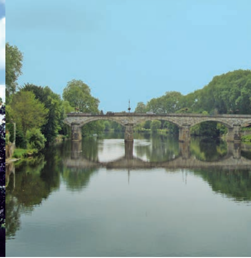
Built of granite ashlar and cut stones, the design of the Pont-Neuf was very wide for the time, so much so that today two trucks can pass each other without difficulty.
