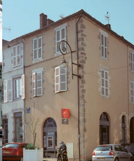
This 18 th century building was the palais de l'élection . Despite many alterations, the building has retained its original openings on the ground floor.
