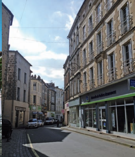
The facades in the Rue du Maquis Foch have been realigned as is shown by the form of the openings.
