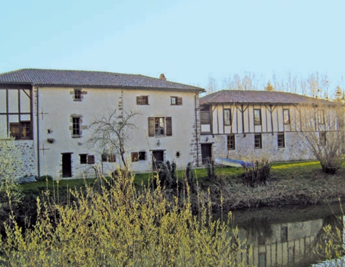
Situated at the confluence of the Vienne and the Issoire, these former tanneries were restored in the early 2000s. Combining stone with timber frames, they still have their cattle horns set in the walls
