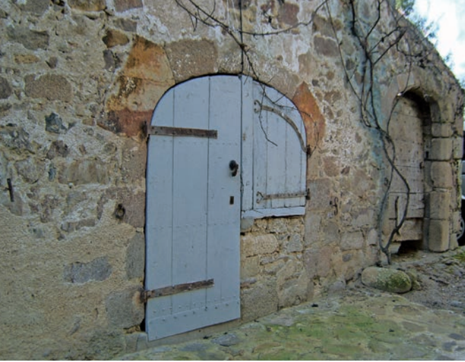
Although it has been reworked, the basket handle shape of this opening reflects the former commercial nature of this building in the Rue Verre de Gris.
