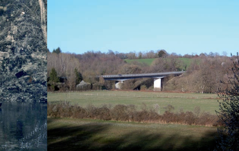
The bypass, constructed at the end of the 1980s, made it possible to stop heavy goods traffic in Saint-Germain by building a new bridge over the Vienne. It is the only bridge built in the 20 th century in the Confolens area on this river.
