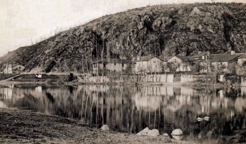
This old photograph shows the tanners' district along the Vienne. The other tanners' quarter was located along the Issoire. The soaking basins were constructed directly in the river.
